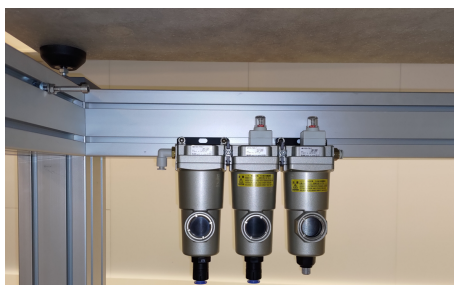
Figure 4-24 Pressurized air filter location
